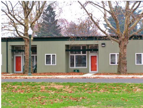
Walnut Street Apartments 117 South Walnut Street, Lititz, PA
